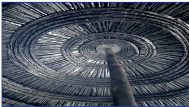
Figure 3: Detail of Coffee House Roof Interior
