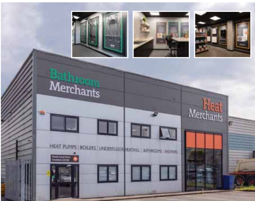
The new Bathroom Merchants' logo featured on the Naas branch facade, with interior insets. https://arrow.tudublin.ie/bsn/vol62/iss5/1
