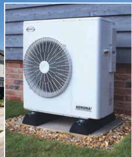
The 6kW Grant Aeronas 3 R32 air to water, air source heat pump installed in all the homes in the Robertstown, Naas development.
