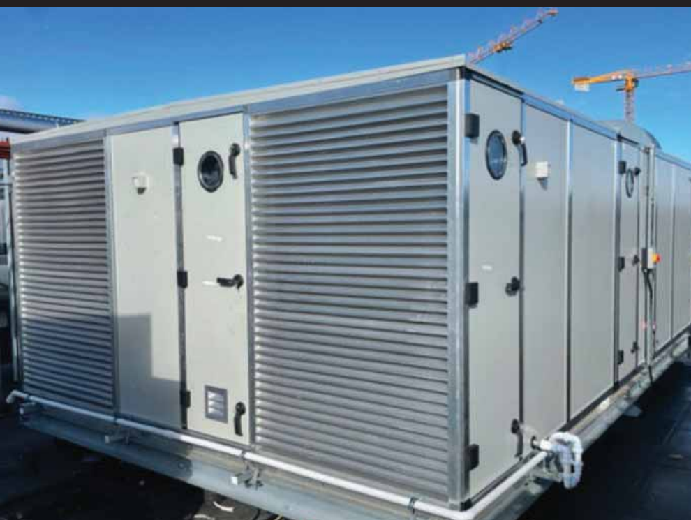
Irish Ventilation & Filtration air handling unit for a pharmaceutical company.
