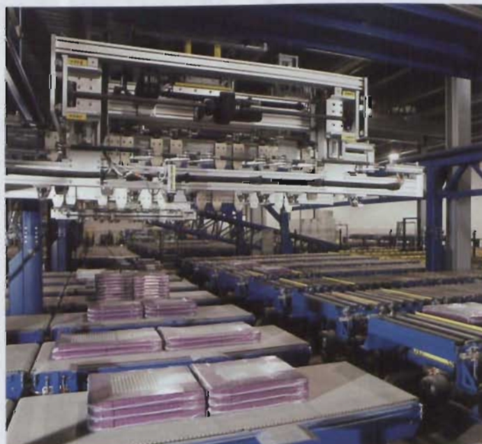
Quinn Radiators' state-of-the-art plant in wales awarded three major quality certs
