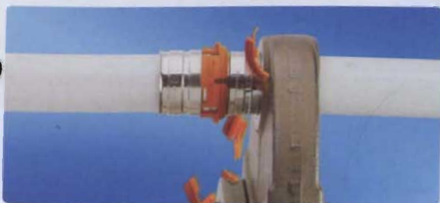
Pressing : the stop ring falls away once the fitting is pressed
