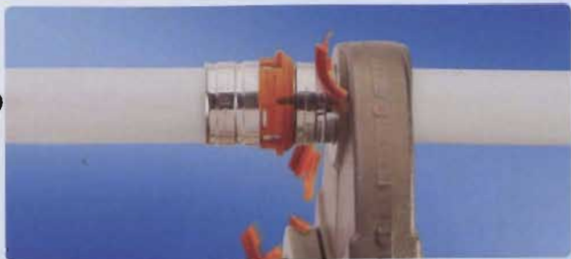
Pressing : the stop ring falls away once the fitting is pressed
