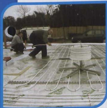
Unipipe underfloor heating
