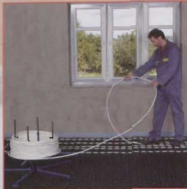
Pipe Laying with Adjustable Pipe Decoiler
