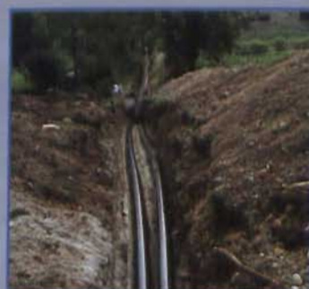
District Heating — pre-insulated pipes. Calpex®
