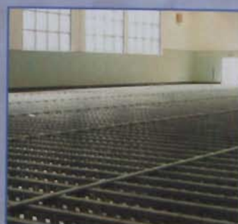
Sprung flooring systems for sports hall. Polysport®
