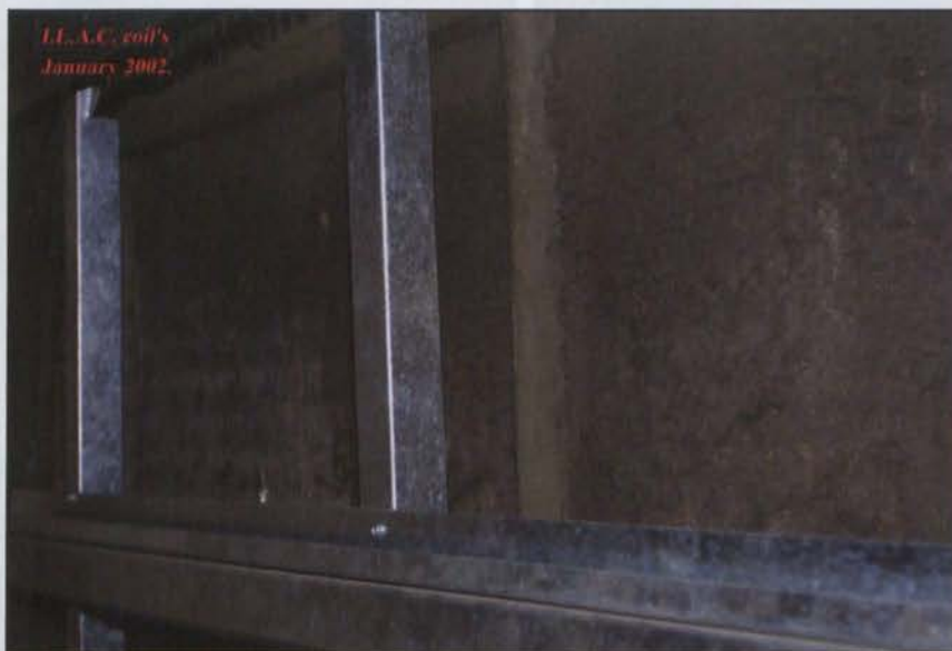
Heating coil in an air handling unit showing obvious signs of filtration neglect
