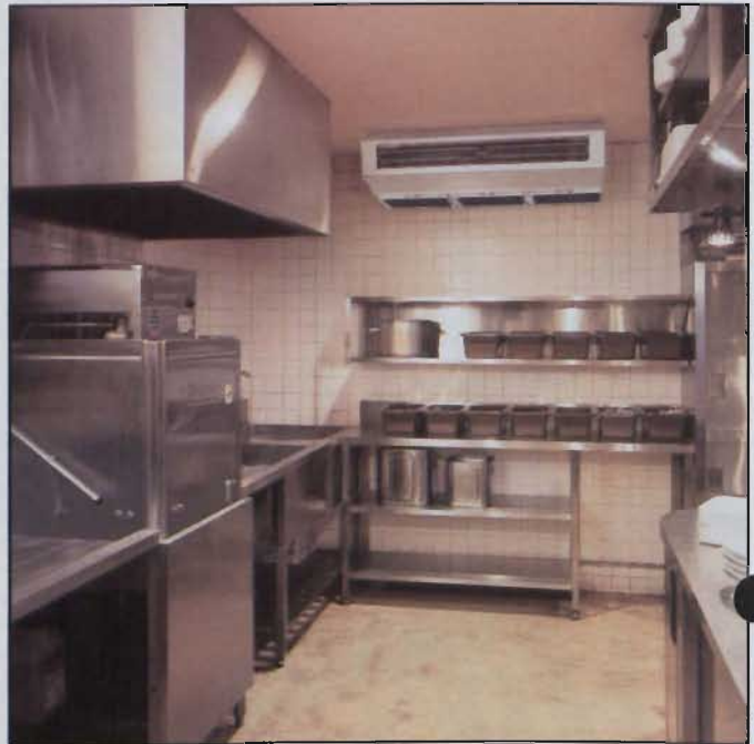
Mitsubishi Electric Mr Slim stainless steel suspended ceiling unit
