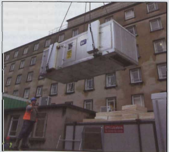
The Air Enterprises AHU unit being delivered to Our Lady's Hospital for Sick Children
