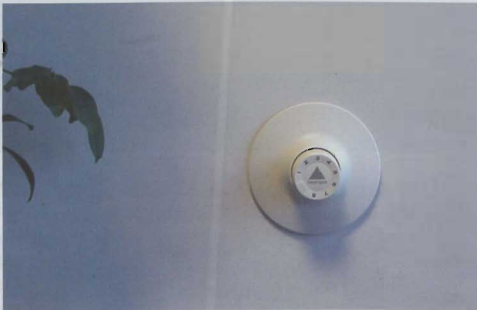
Danfoss FHV valves are fitted with either FJVR or RA2000 sensor elements
