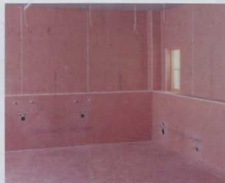
The units are now ready for cladding.
