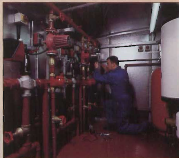
Packaged boilerhouse being pre-piped and pre-wired with TAC controls
