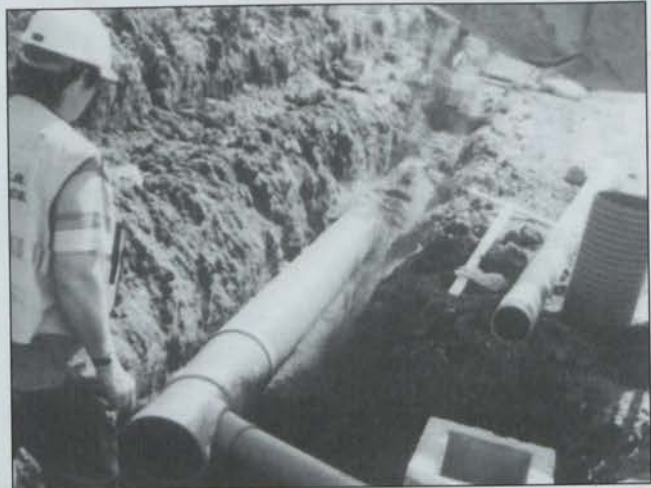
MFP Sales' Quantum technology is a PVC-u twin-wall manufacturing process combining corrugated outer wall with a smooth inner bore to give strength, hydraulic efficiency, and lighter weight than comparable products.
