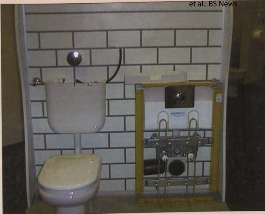
Custom-made display showing the internal workings of the DAL-RAPID "S" system
