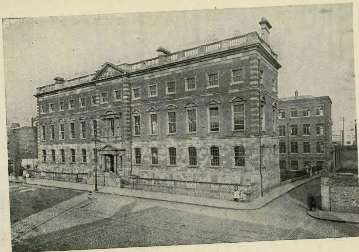
BOLTON STREET TECHNICAL INSTITUTE.
