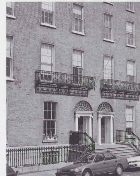
DIT Fitzwilliam House (Central Office).
