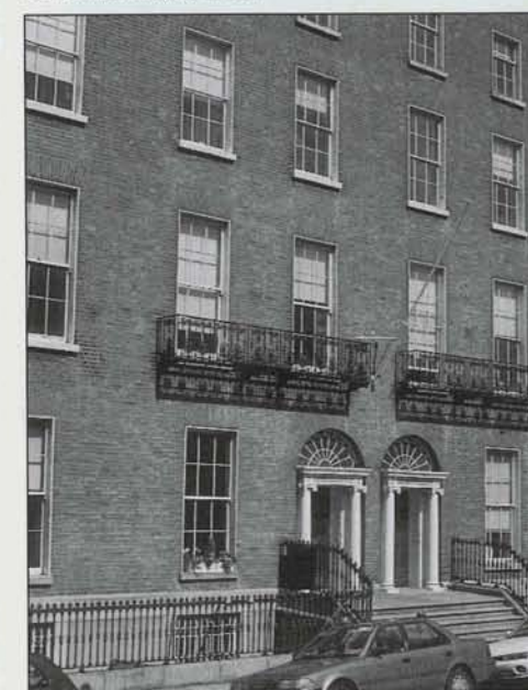
DIT Fitzwilliam House (Central Office).
