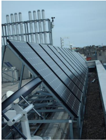
Fig. 7 Anemometer mounted on Focas building, DIT, Kevin St.
