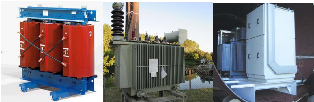
FIGURE 3.5 LEFT TO RIGHT: DRY TYPE, OIL FILLED AND SYNTHETIC FLUID FILLED (COURTESY PELAMIS WAVE POWER LTD.) TRANSFORMERS
