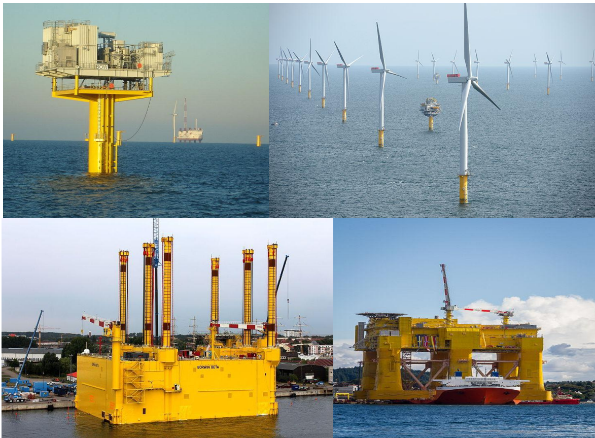
FIGURE 3.34 OFFSHORE SUBSTATIONS (FROM TOP LEFT CLOCKWISE) – BARROW (2006, 450T, 90MW, COURTESY WIKICHOPS), SHERRINGHAM SHOAL (2011, 875T, 316MW), BORWIN BETA (HVDC – SELF INSTALL) (2014, 10,000T, 800MW, COURTESY WAERFELU). DOLWIN BETA (HVDC – SELF INSTALL) (2014, 20,000T+, 900MW, COURTESY STEN DUELAND)
