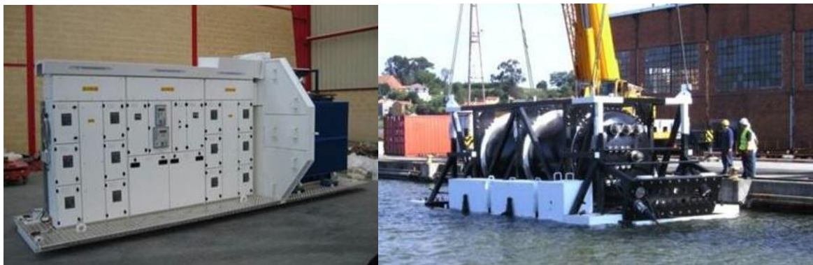
FIGURE 3.28 OPT'S UNDERSEA SUBSTATION POD (USP) INTERIOR SWITCHGEAR (L) AND INSTALLATION (R) (SOURCE: OCEANPOWERTECHNOLOGIES.COM)
