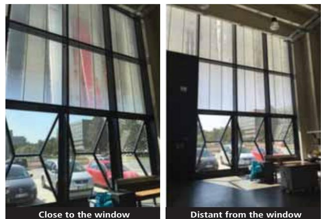
Figure 4: Interior projection of daylight by a prismatic glazing at TU Darmstadt, Darmstadt, Germany.
