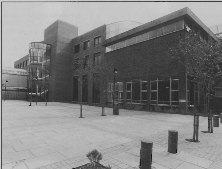
Kevin Street College Extension 1987. View from Internal Courtyard.
