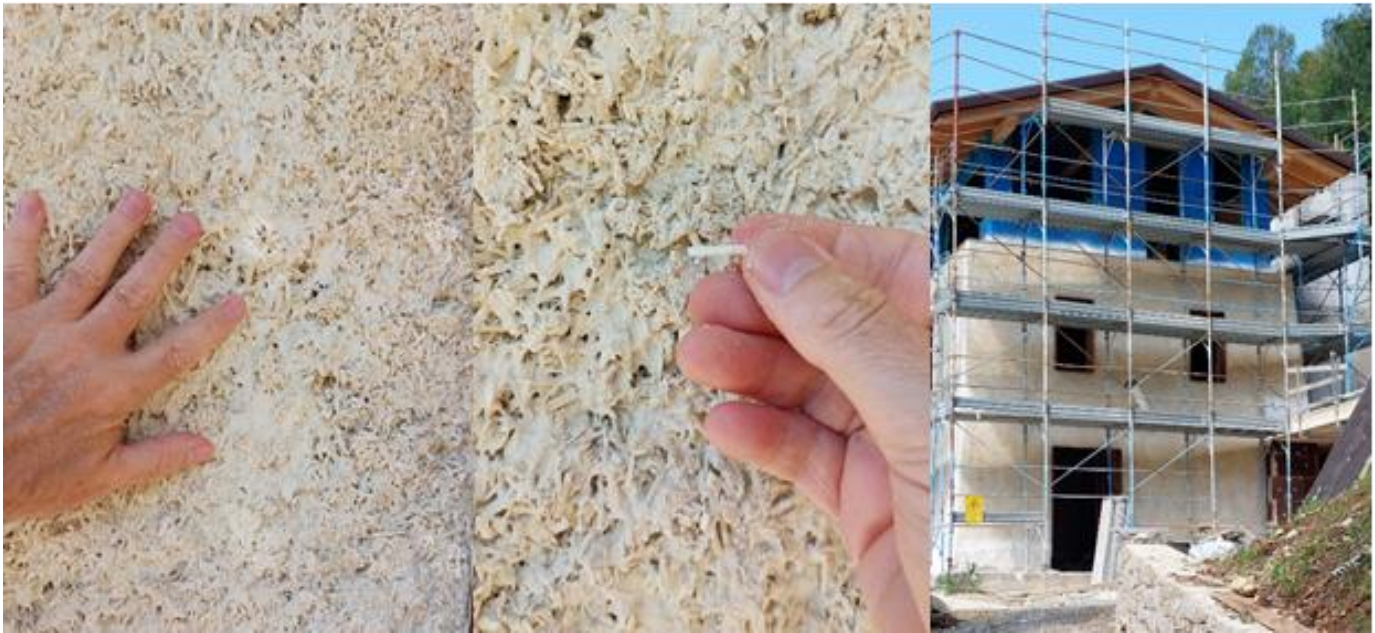
Figure 8: Showing hempcrete spray applied to existing masonry wall in rural house renovation. Senini-Tecno Canapa northern Italy [Source Author].
