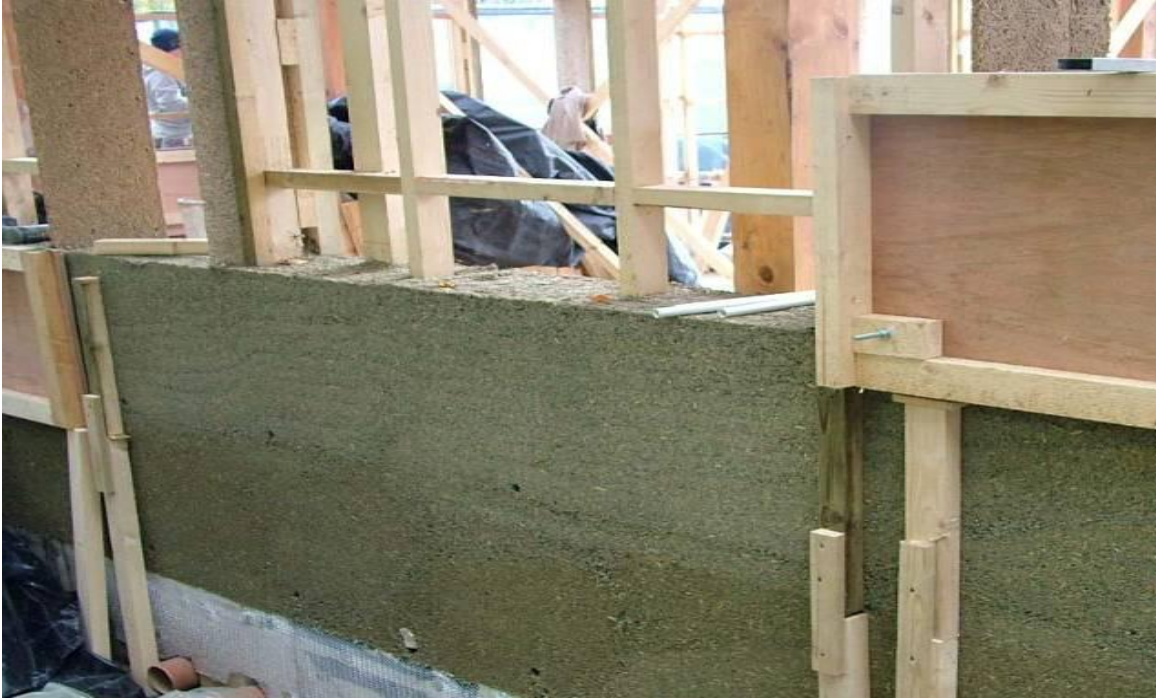
Hemp Lime wall infill in timber frame after striking of shuttering: Photo BESRaC
