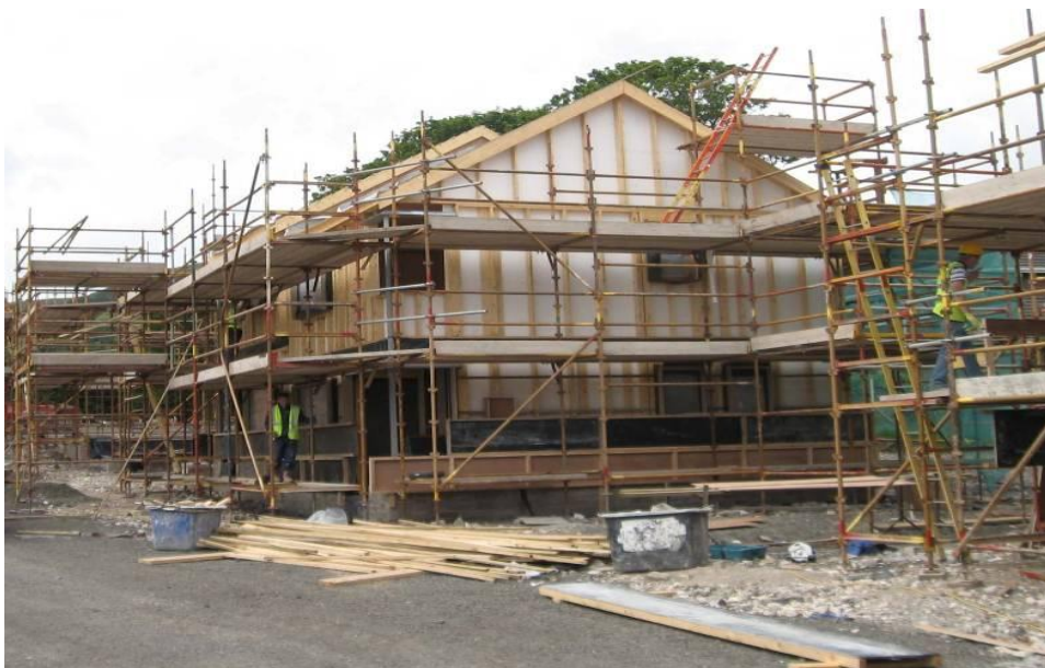
Hemp Lime infill to timber frame semi detached housing units at Carnlough, Co. Antrim, Northern Ireland. Early shuttering above and later pre rendering stage below. Photo BESRaC / Tom Woolley
