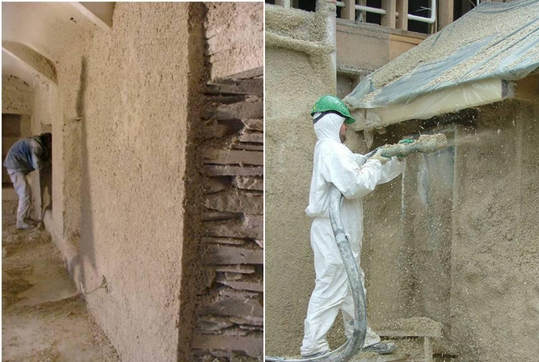
LHS Internal Hemp Lime application to an old stone wall Photo Steve Allin
