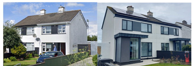
Fig 1. LHS photo of existing demonstrator case 1970’s two story semi detached houses. RHS photo of completed front elevation with circular / modular wall panels and extension ‘pod’. Source Author.
