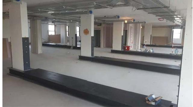
Fig. 11: Steel Supports for Shelving (photo: Catherine Cooke, 2020)
