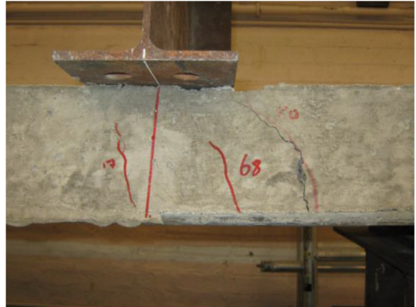
Diagonal Shear cracks – Right hand side
