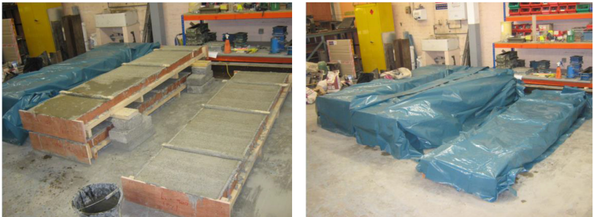
Figure 4 (a) Cast composite slab and (b) curing under polythene
