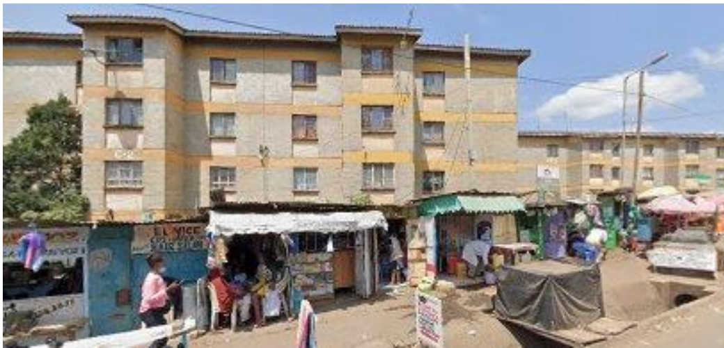
Figure 49. A high-rise building constructed as part of the Nyogo high-rise project
