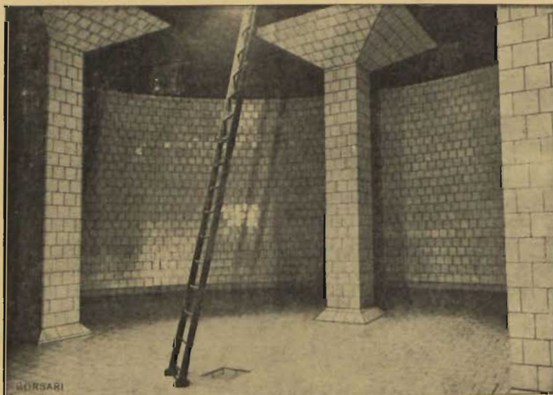
UNDERGROUND FUEL OIL STORAGE TANK 70,000 GLS. (DUBLIN)
