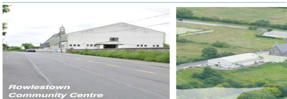
Figure 2. View of Existing Building
