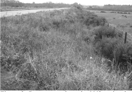
Figure 2. Rampart road on the N62 national secondary road, County Offaly, Ireland.
