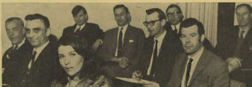
● Members of the Organising Committee of the Heating and Ventilating Exhibition, 1969.
