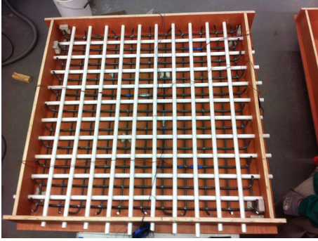
FIGURE 11: PVC duct locations prior to casting.
