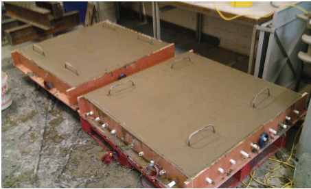
FIGURE 12: Lifting eye positioned during casting.
