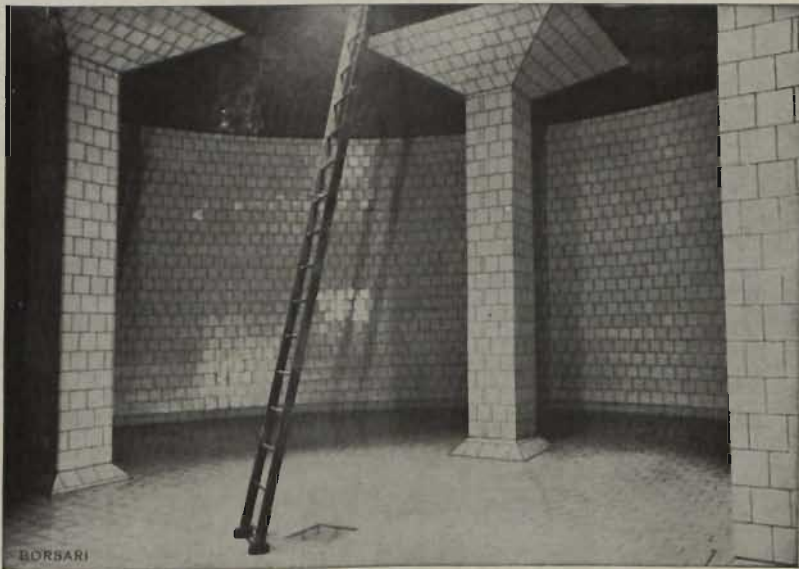
UNDERGROUND FUEL OIL STORAGE TANK 70,000 GLS. (DUBLIN)
