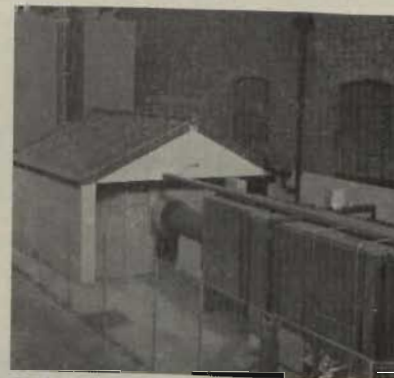
● General view of cooling tower test centre showing, on left, the twin cooling towers and, on right, the air conditioning equipment.
