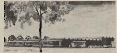
● THE new Scanglo plant
