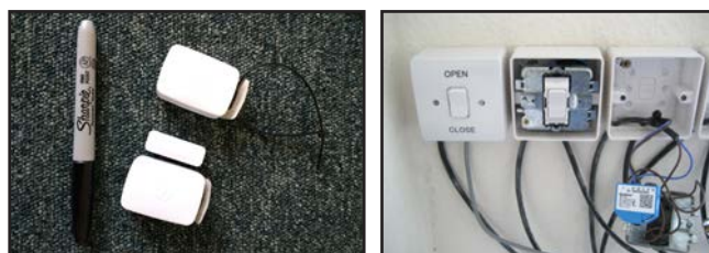
Figure 10. Left – wireless temperature sensor which relayed room air temperature data to the controller. Right – wireless receiver embedded behind each window switch which controlled window opening.
