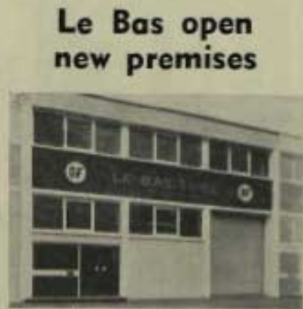
● The new Le Bas Tube Co. Ltd. warehouse and sales office at 472 Shore Road, Belfast 15.
