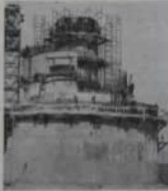
The now familiar bulk of the Kish light under construction.
