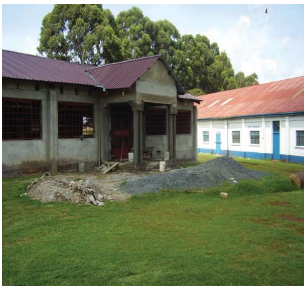
Image 7 New library under construction
