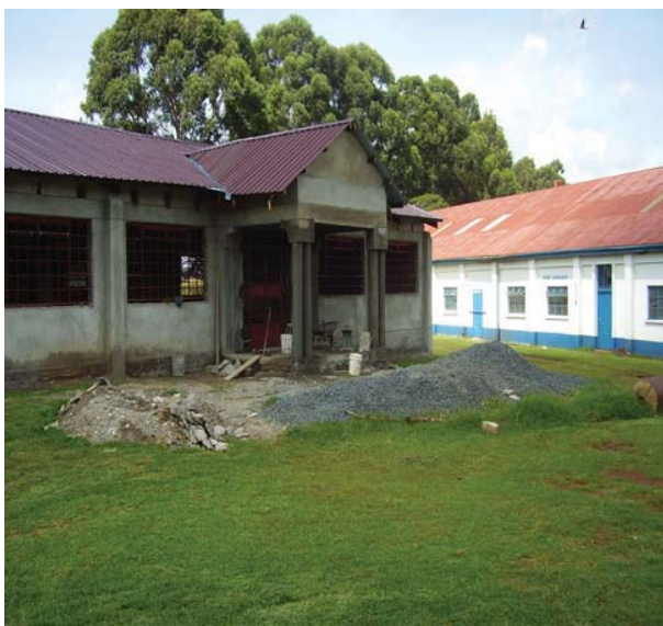
Image 7 New library under construction
