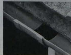
4. The silt bridge in place sealing the joint and preventing the entry of sand and silt.
