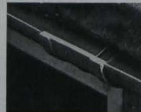
3. Silt bridge being snapped into position.
