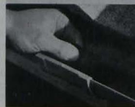
2. Gutter snapped into position either side of projecting tongue which allows automatically for expansion.
