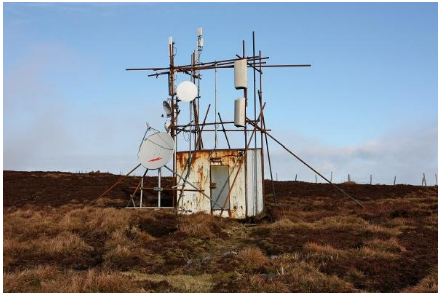
Figure 9-2: Deflector site in Coumaraglin/Comeraghs, 2010 [Moun2010].
