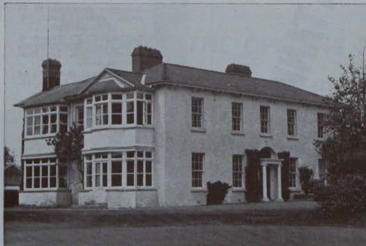
A Harper Meehanite 300,000 Oil-fired boiler is now heating Ballygowran House, Maynooth, Co. Kildare.
