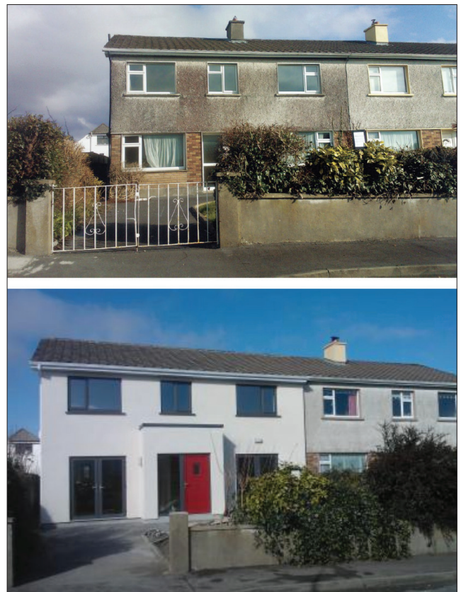
Figure 1. Case-study building — the existing dwelling prior to, and after PH retrofitting works (McGuinness, 2014).
