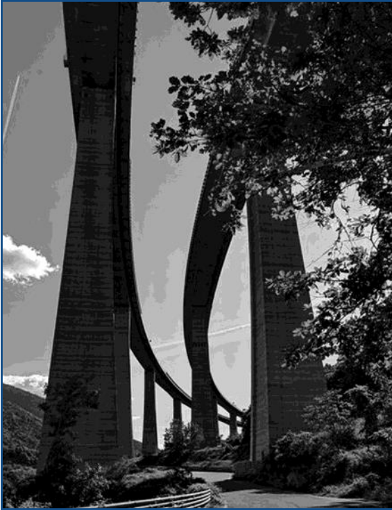
Figure 12. A motorway viaduct in the upper part of the Susa Valley.
