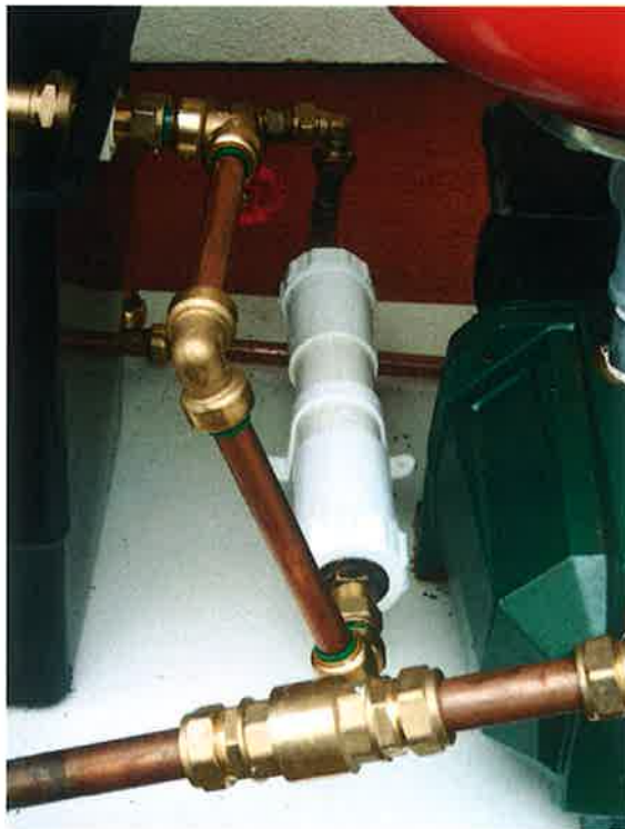
Figure 5.4 Modified Carbon Filter in Revised Position.
