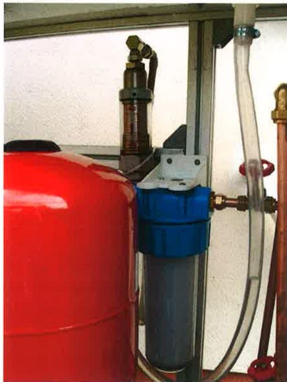
Figure 4.2 Flow Control Valve and Flow Meter.
