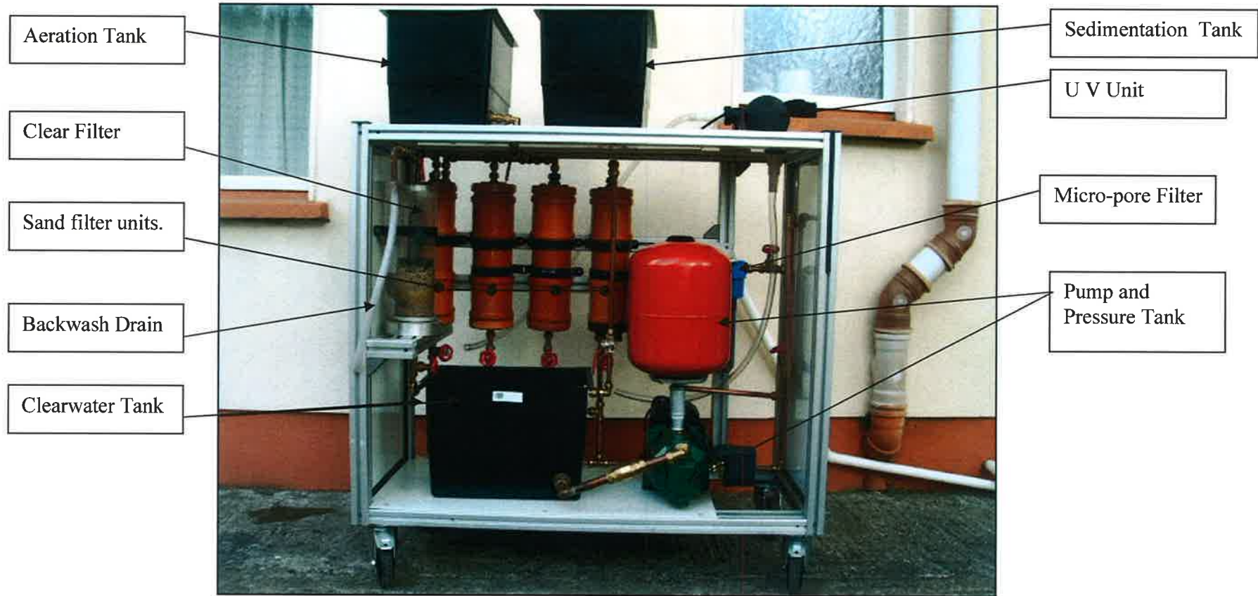
Figure 4.6 Labeled Image of the Laboratory Treatment Unit.
