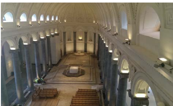
Figure 12: Lighting installed and operating.
