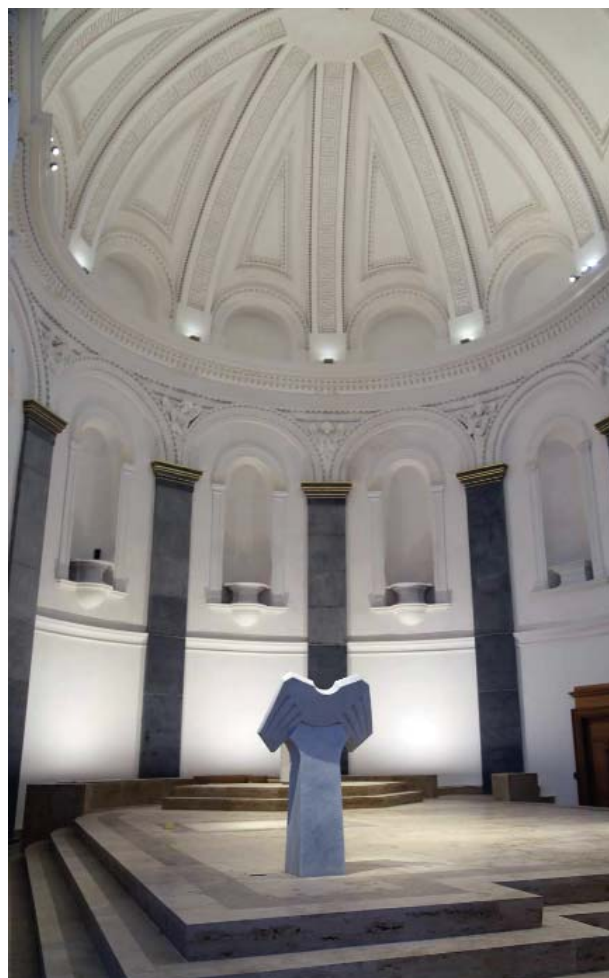
Figure 9: The Ambo during commissioning of the lighting.
