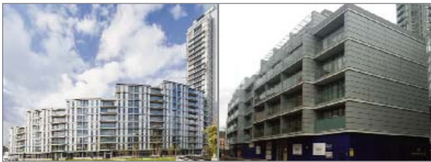
Figure 1: The Seager Distillery site and Norfolk House.
