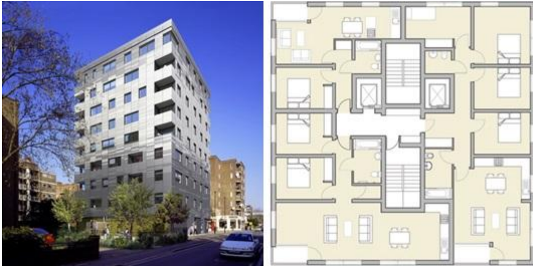
Figure 8. Murray Grove timber residential building, Hackney, London.
