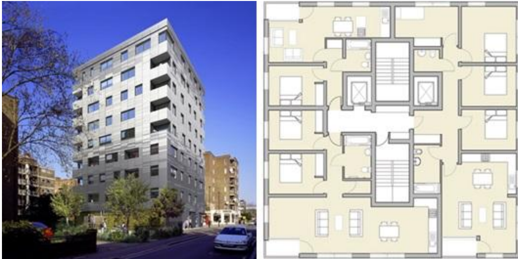
Figure 8. Murray Grove timber residential building, Hackney, London.
