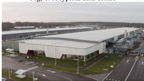
Fig. 1. A typical data centre
