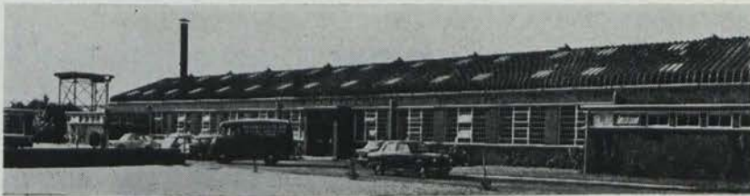
Shown here is the extended Santry factory of Sanbra Fyffe Ltd., which was officially opened this month by the Minister for Industry and Commerce, Mr. J. Lynch, T.D.
