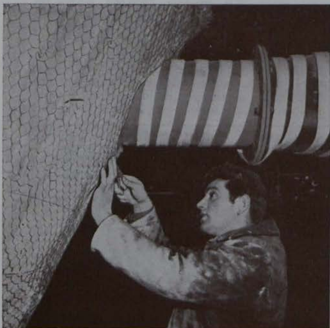
Vessel heated by Isopanel and pipes by Isotapes
