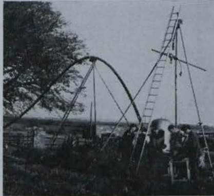
The giant length of H.D.P. is lowered into the well.
