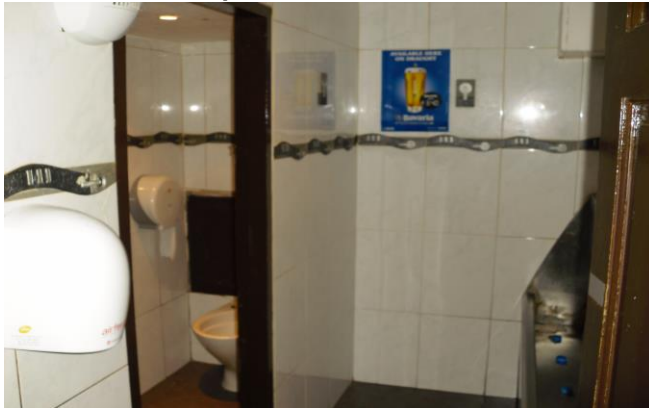
Case example: Toilet Area.
