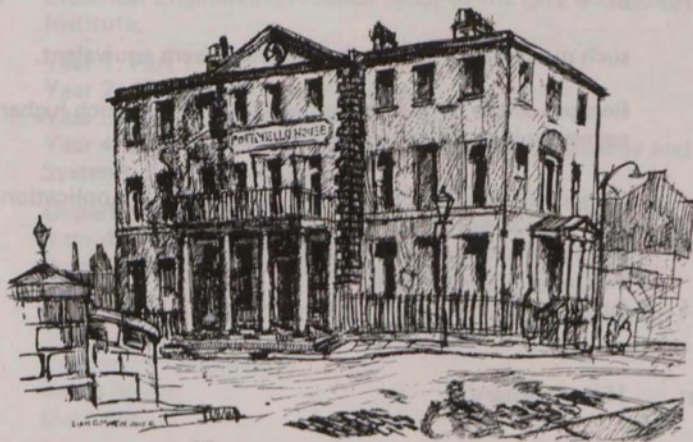
PORTOBELLO HOUSE, PORTOBELLO HARBOUR
